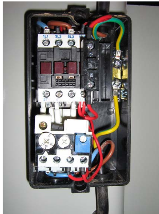
Figure 16 & 17 Single Phase DOL starter that is still based on a three pole switch inside.
