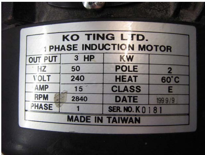
Figure 2 A typical single phase motor rating plates (Taiwan & Europe)
